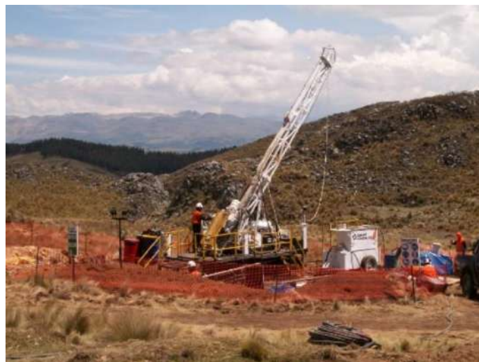
Figure 6.10 Estrella core drilling at Colpayoc (Yanacocha Mine in background).
